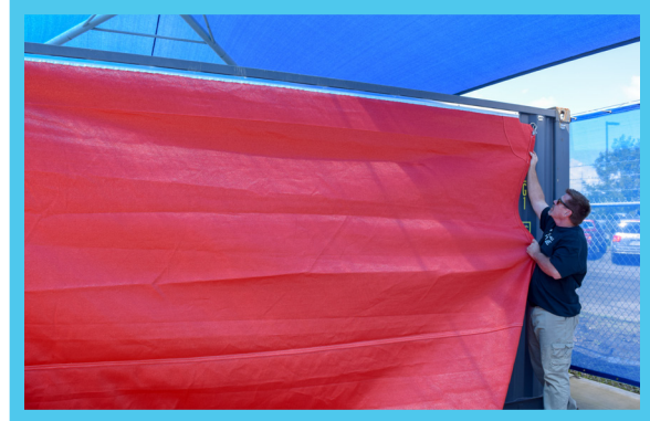
Guide the Keder through the Channel
