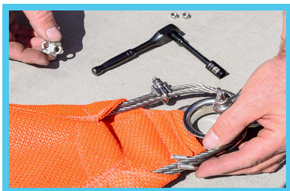
Place Cable Clamps on either side of the D Ring
