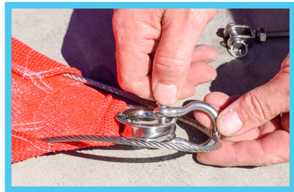
Connect D Ring Thimble & Bow Shackle
