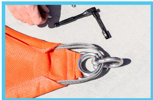
Both cable ends should be tucked into the pockets and looped around the D Ring and Thimble
