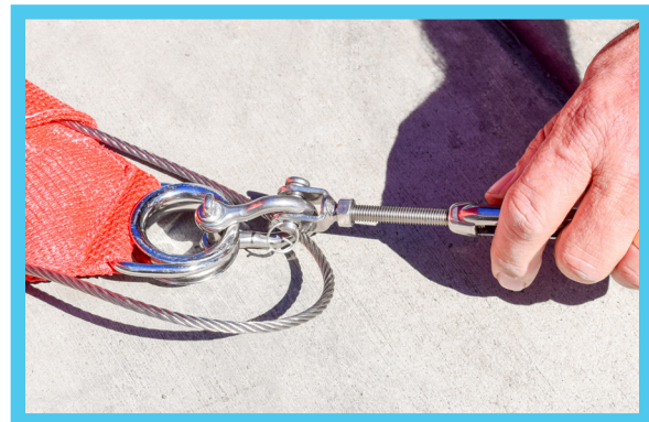
Connect Bow Shackle & Turnbuckle
