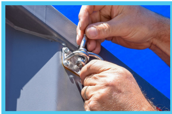
Connect Bow Shackle to Attachment Point
