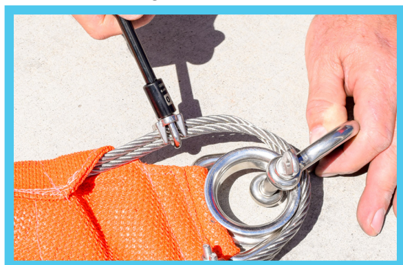
Tighten Cable Clamps
