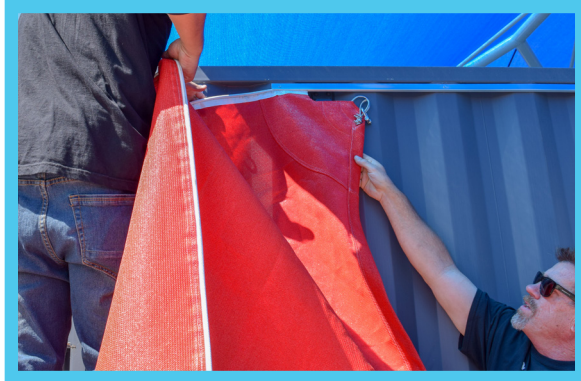
Feed one end of the Keder through the C-Channel
