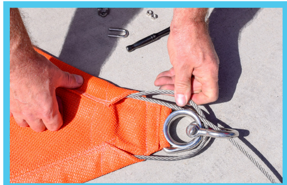
It should loop around the D Ring and Thimble
