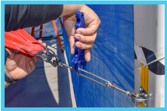
Tighten the Body of the Turnbuckle
