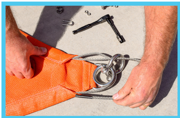
Feed other Cable End into pocket
