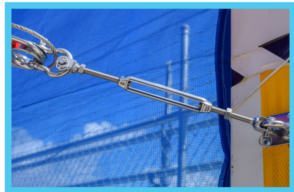
Connect Turnbuckle to Attachment Point
